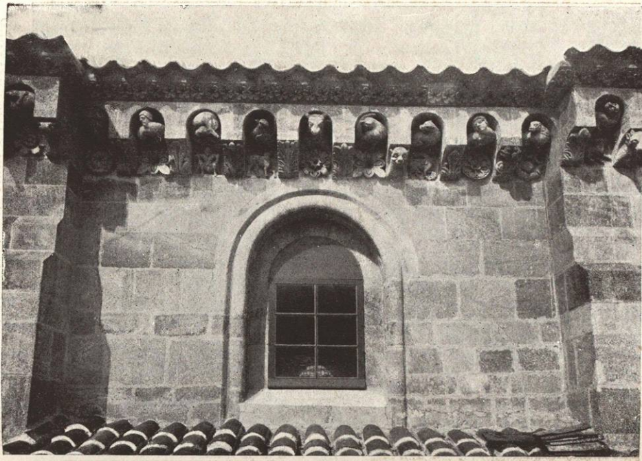
BASILICA OF SAN VICENTE. — DETAIL OF THE MIDDLE CORNICE, RESTORED AVILA
