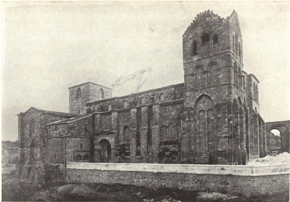
BASILICA OF SAN VICENTE. NORTH FAÇADE AVILA
