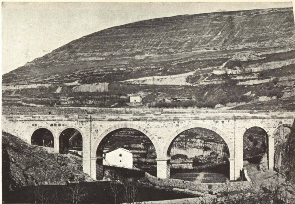
AQUEDUCT OVER THE RIVER CASTILLA SEGOVIA
